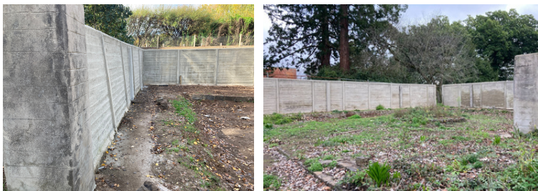
Buninyong Botanical Gardens baths restoration works.
