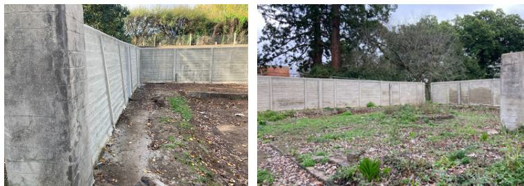
Buninyong Botanical Gardens baths restoration works.
